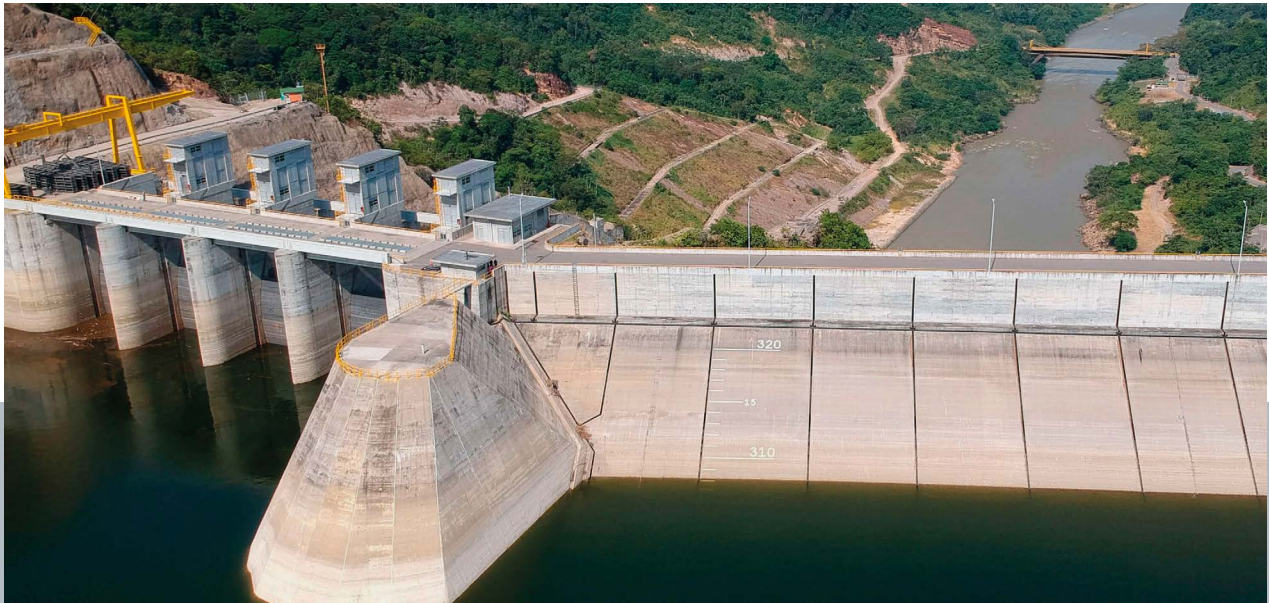
Sogamoso Hydroelectric Plant.
